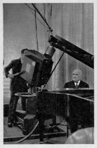
Visual action, recorded by the camera, and sound, picked up by the microphone, are blended to form the complete televised program
