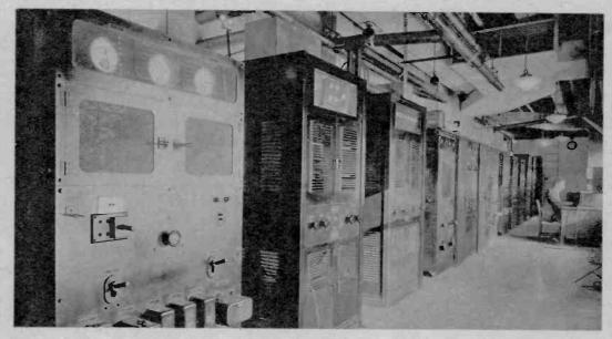
Half the units shown above are audio (sound) transmitters, half video (pictures). In the pipes, audio and video signals are combined in an antenna filter. Thus simultaneous sound and picture transmission is possible. Program is piped to antenna—then into air
